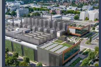
Data Centre, Substation Infrastructure Goedman (Frankfurt)
