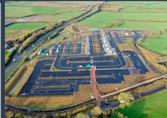
A40 Infrastructure Upgrade Oxfordshire County Council
